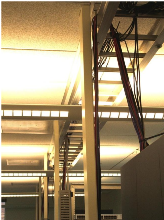
Illustration 4: The "ladder" carrying network cabling between rows of workstations. Note the bundle of cables rising obliquely from the server rack (right foreground) to the ladder, and vertical bundles of cables running from the ladder down to the trough below (not shown).
