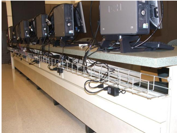
Illustration 3: View of a row of workstations, showing the wire trough for laying network cabling.
