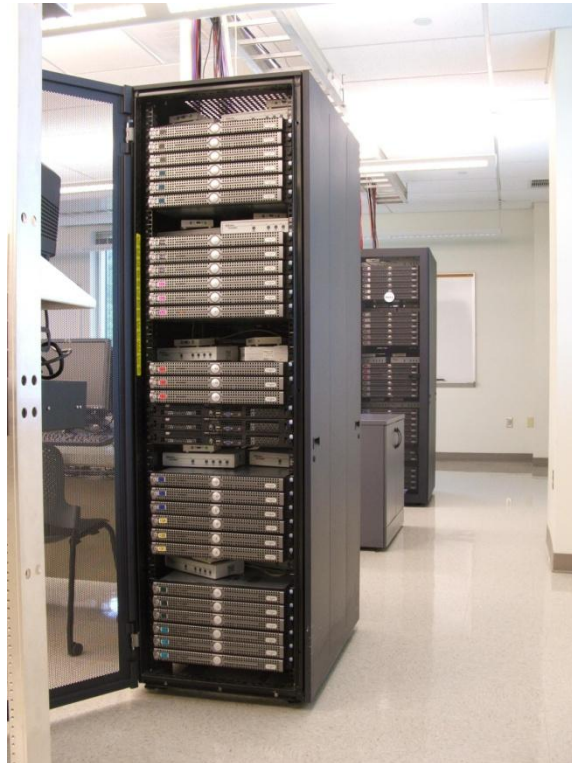
Illustration 5: Rack of 30 1-U servers. Note the boxes of KVM switches above each cluster of six servers. The bottom three servers in the middle cluster have their escutcheons removed to allow access the optical drives and USB ports.
